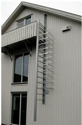
Pull out the locking/release pin (this makes the ladder burglarproof). Open the ladder and it's ready for use.
